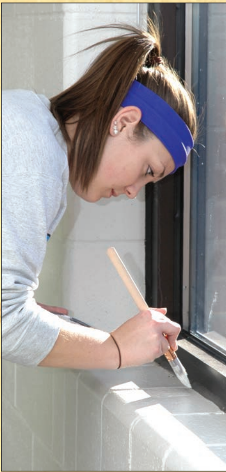
Steady hand: Wayne State College's Kristyn Huelskamp touches up fresh paint on a windowsill at C.L. Jones Middle School in Minden.
